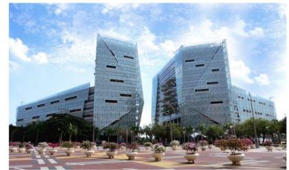
According to the annual windrose diagram of Putrajaya, most winds come from the south and east-north-east. With that being said, Suasana PjH 2C5 takes advantage of that by using the winds to form a venturi effect by creating a gap between the architecture.
